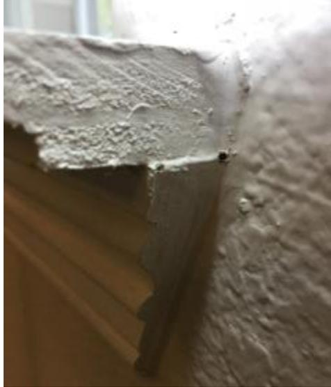
We frequently find a series of these holes, or “breakouts.” They may follow each other in a straight, vertical line. Following the grain of the stud, they may curve toward the sheet rock and go through the same procedure of tunneling through it and plugging the opening.
