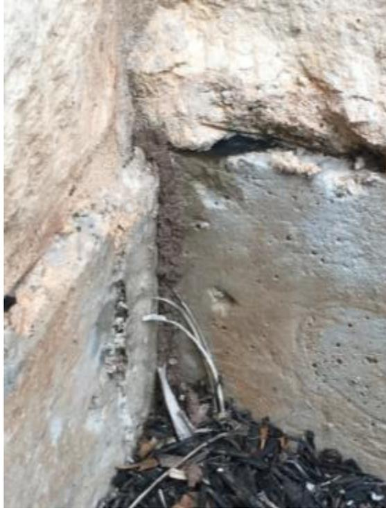
Often, we find these tubes on slab foundations. It is not uncommon for the shelter tube to be visible from the soil level to the lowest course of bricks or the wood siding. The mortar at the lowest course of bricks or a crack in the concrete slab may provide sufficient space for termites to enter a structure. Any penetration of the slab such as a bath trap or plumbing penetration may provide an avenue of entrance for termites.
