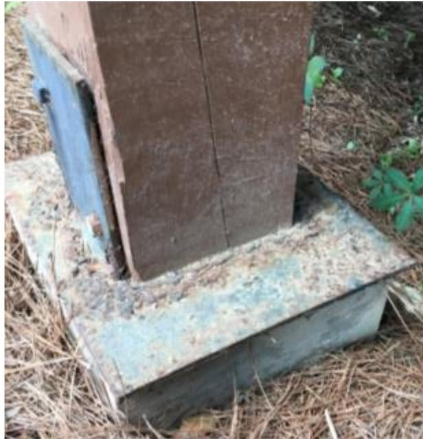
The edges of the exclusion device are bent down slightly, so that termites cannot build a tube around that edge. These shields can be installed during construction or retrofitted. This type of treatment is not practical in most cases and has extremely limited value.
