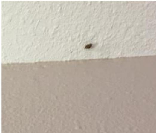
Once you have inspected the interior walls over any cold joint or crack and carefully inspected the interior walls on the perimeter of the house, move to the bathroom area. I say "area" because evidence of termites entering through the bath trap may appear in an adjoining room.
