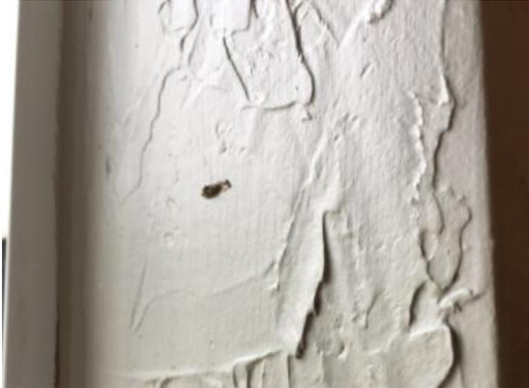
Sheetrock, the most common interior product in our houses, has paper on both sides. As termites work through the studs in the wall, they follow the grain of the wood. The grain often curves toward one side of the wood. This leads the termite workers out of the wood and into the paper backing on the sheetrock.
